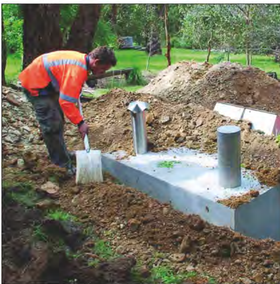
Compacting by hand.
