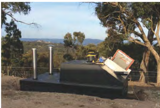
12 PERSON UNIT INSTALL
