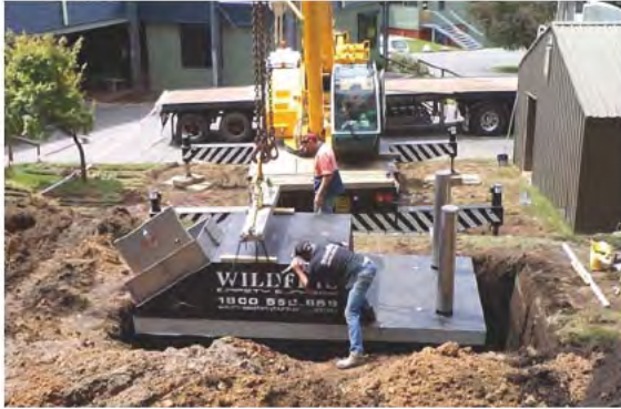
12 PERSON UNIT INSTALL
