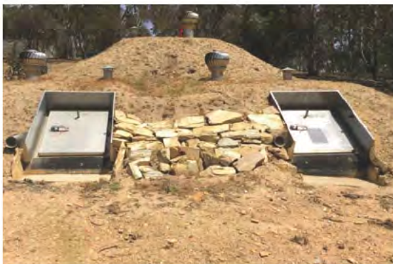
CONNECTED BUNKERS INSTALLED
