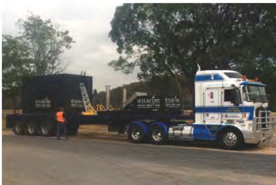
12 PERSON UNIT DELIVERY & INSTALL
