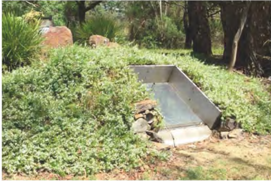
12 PERSON UNIT INSTALL
