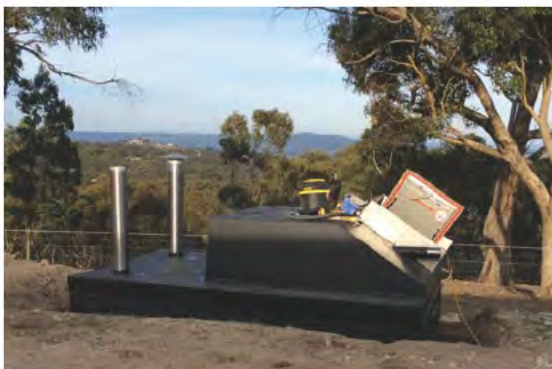
12 PERSON UNIT INSTALL
