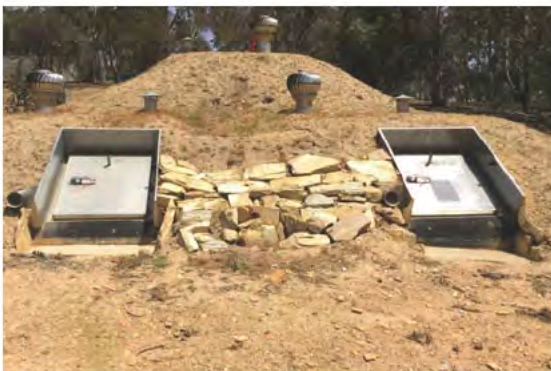
CONNECTED BUNKERS INSTALLED
